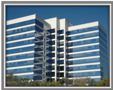
BSK performed complex environmental engineering services turning this former Brownfields site into 3,000,000 square feet of developed land.
